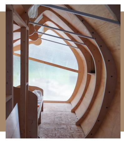
The construction process also involved integrating DfMA techniques to streamline the monocoque ribbed system's fabrication and communication processes.
