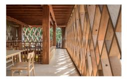
All wooden elements of this project were prefabricated at the factory and then transported to the site to minimise noise and dust. This process also mitigated any damaging impact to the surrounding environment on-site. More precision went into the cutting of the materials in the factory as it was carried out by trained professionals under higher safety standards which ultimately led to a safer/easier construction process.
